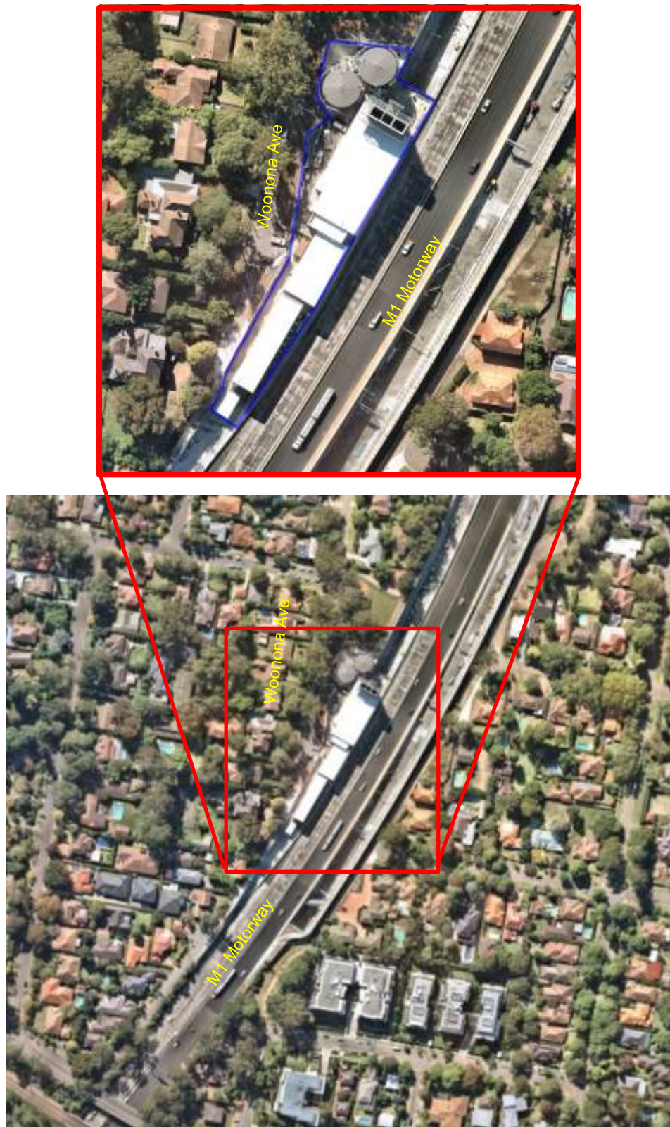
Figure 2: Northern Ventilation Outlet
